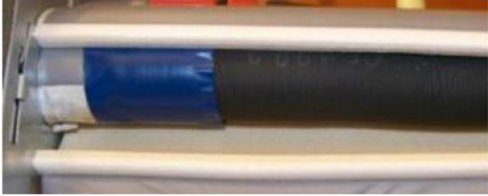
Insulate around flare nuts
