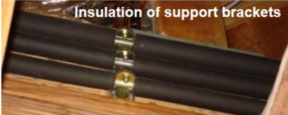
Tighten brackets so that they hold pipes in place but still allow for expansion
